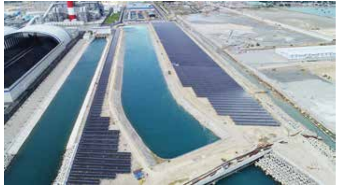
Solar Power Plant at Vinh Tan Power Complex
