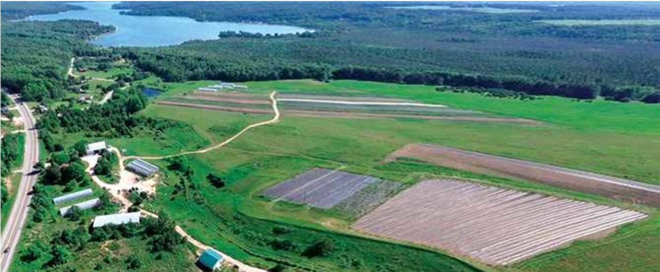
Aerial survey 500m above 220kV Thanh My - Duy Xuyen Transmission Line
