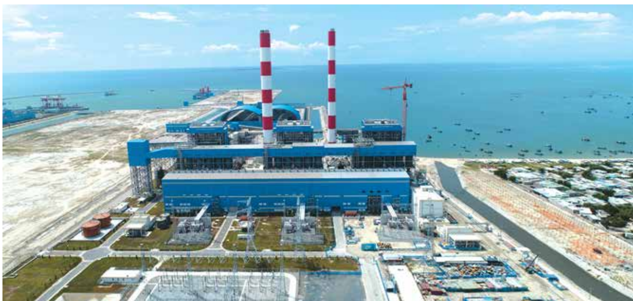
Vinh Tan 4 and Vinh Tan 4 Extension Power Plant Projects
