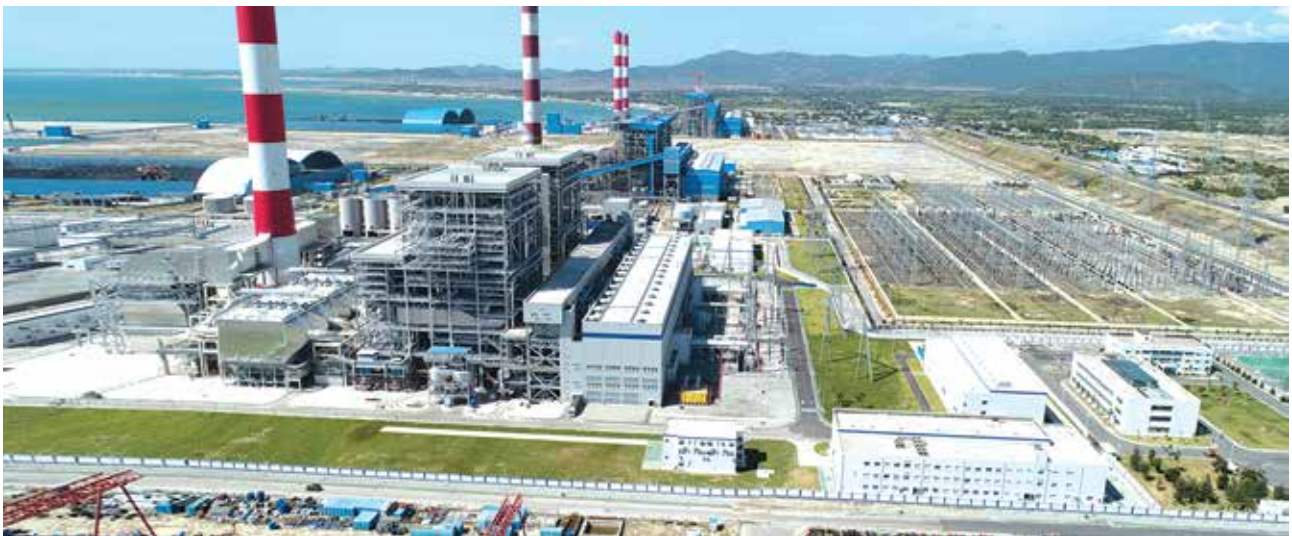
Vinh Tan Power Complex
