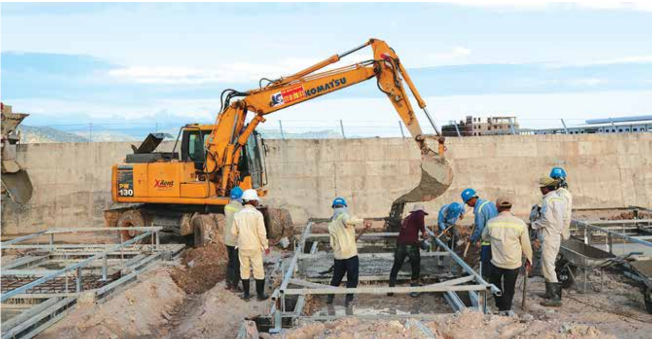
Construction foundation of Solar Power Plant at Vinh Tan Power Complex
