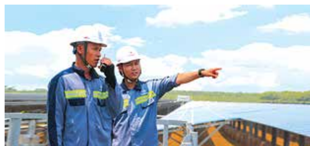
Operation takeover of Dau Tieng 3 Solar Power Plant
