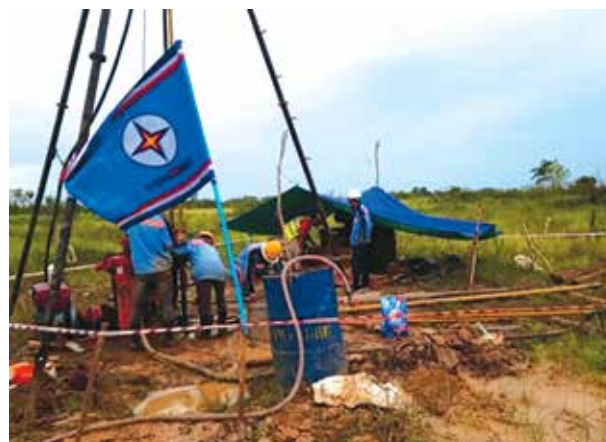
Survey drilling at New Phnompenh Airport Project in Cambodia
