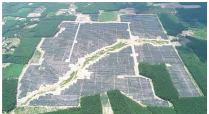
Son My 3.1 Solar Power Plant
