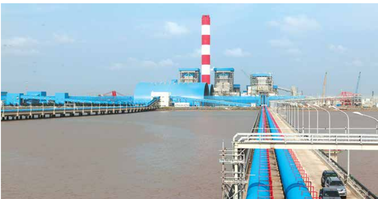
Duyen Hai 3 and Duyen Hai 3 Extension Thermal Power Plant project
